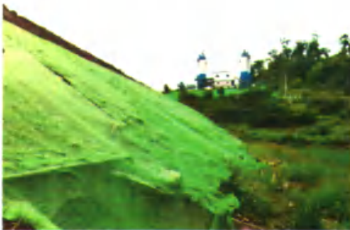
裸露地表临时苫盖
